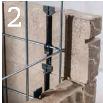
2 Use connector to attach veneers to grid
