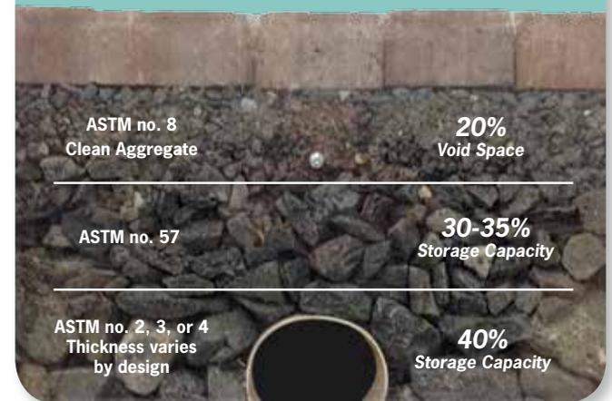
“The stone bed underneath the pavers acts a stormwater filter to slow down runoff, allowing it to soak into the ground rather than carrying pollutants into adjacent water sources. The pavers also have an overall aesthetic appeal; they look better than conventional paving solutions.”
